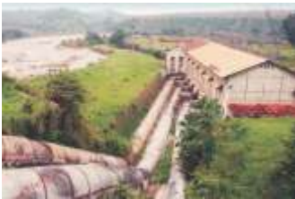
SANGA POWER PLANT
