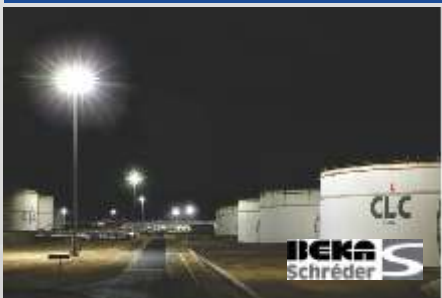
Portholes, high ceilings, low ceilings, classified luminaires and industrial fluorescent lights.
