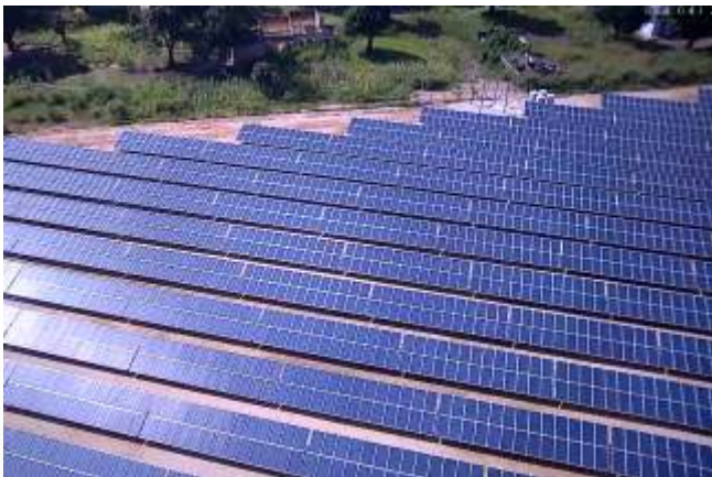
AERIAL VIEW OF THE POWER PLANT
